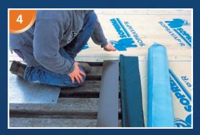
Where the ends of the rolls overlap (15 cm / 6 in.), install a metal plate\* to support the end laps between the flutes and ensure a perfect end lap seal. \*Format: (15 cm x 106 cm / 6 in. x 42 in.)
