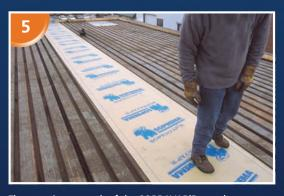
The superior strength of the SOPRAVAP'R membrane provides added protection against heavy work crew traffic during installation. The nonslip surface allows for safer foot traffic.
