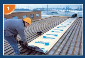
Roll out the SOPRAVAP'R membrane on the clean, dry metal deck. Peel back the first metre (3 ft.) of the silicone release film and adhere the membrane in place.
