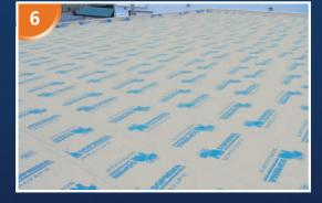
Once the installation has been completed, the SOPRAVAR'R membrane provides temporary protection against inclement weather.
