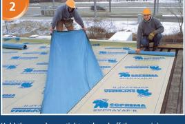
Hold the membrane tight and peel off the remaining silicone release film diagonally.
