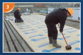
Install adjacent rolls of membrane in the same way, taking care to overlap the longitudinal joints by 7.5 cm (3 in.). Use a roller to seal the joints.
